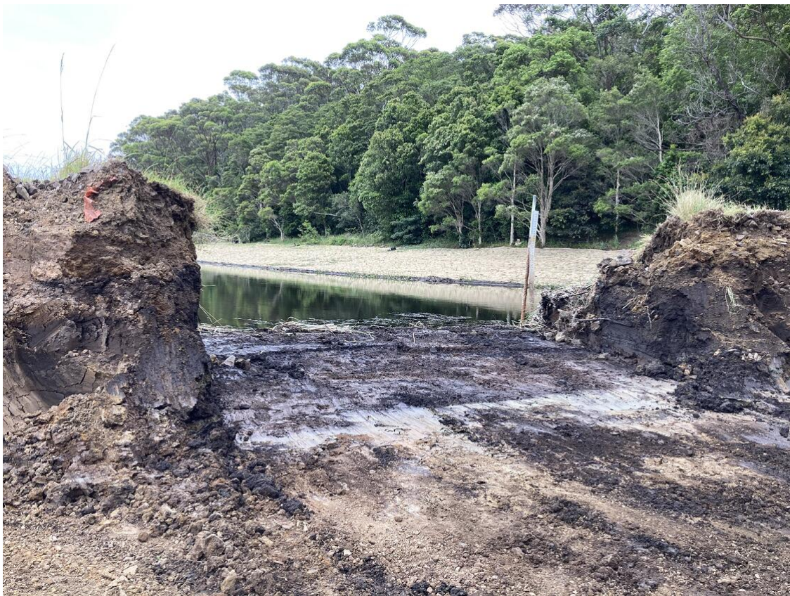
A cut was made in Blackbutt Dam's embankment wall to install a low flow pipe.
